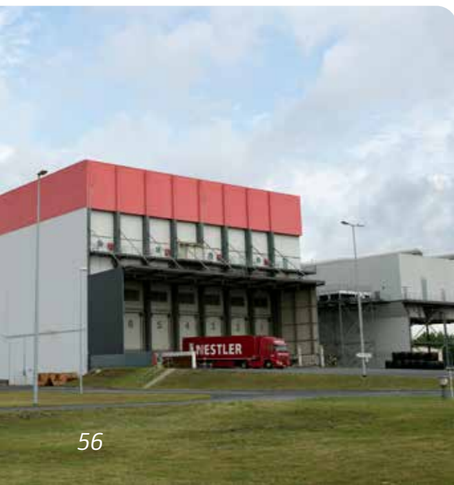
Energy optimisation at the Großräschen site
